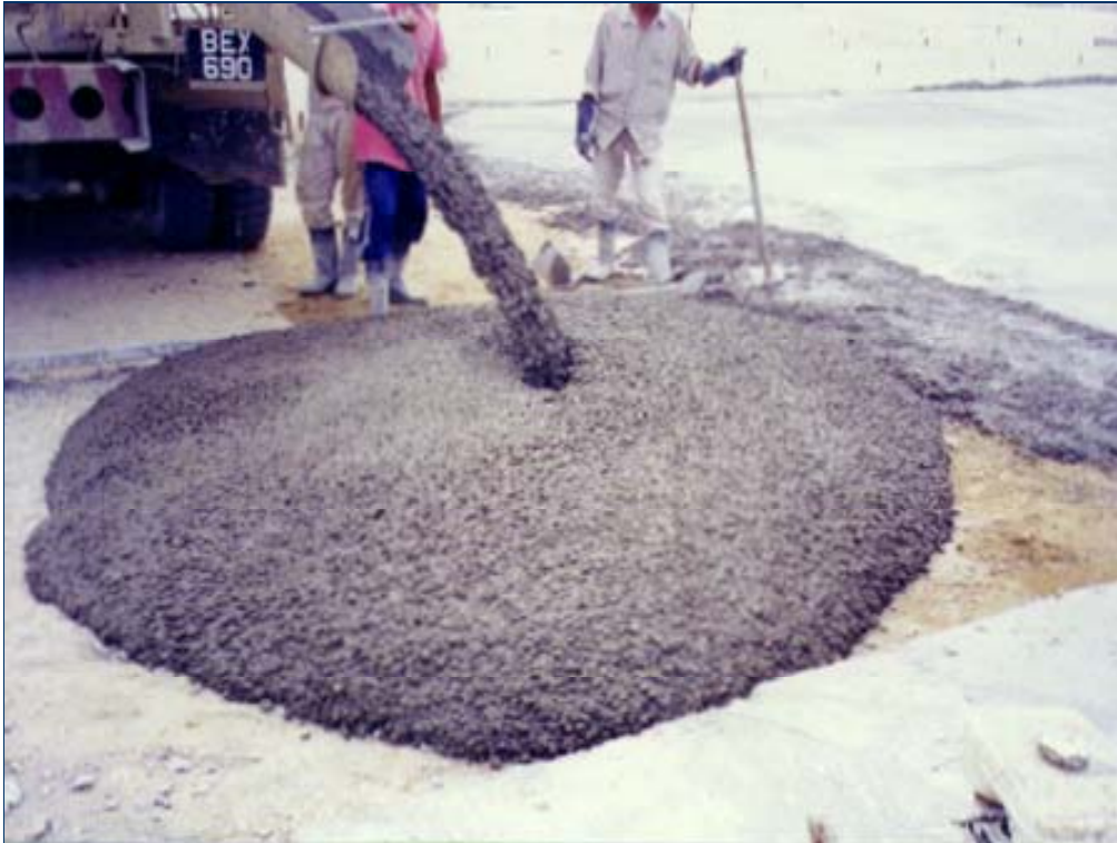
Fig 1 : Direct discharge of concrete
